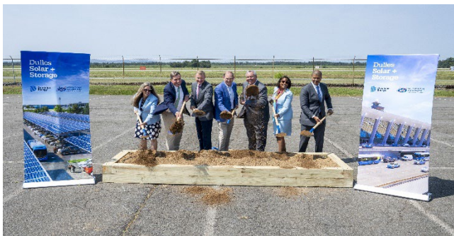
Figure 3: Airports Authority, Dominion Energy Break Ground on Solar and Energy Storage Project at Dulles Int'l. Airport
